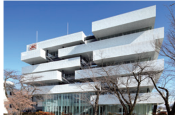
Advanced Technology Center (Nagano)
