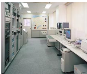
Komagatake Warning and Evacuation System (Japan)
