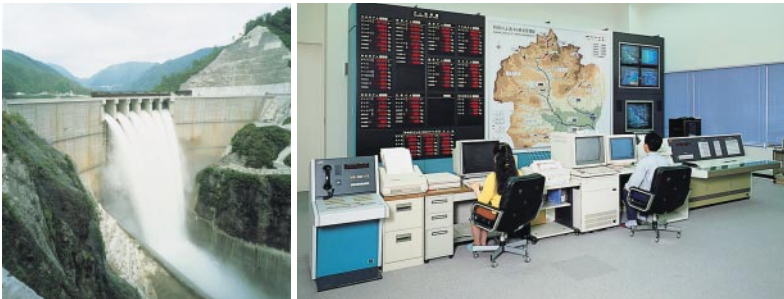
Integrated dam management system
