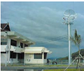
Bili Bili Dam Telemetry System (Indonesia)
